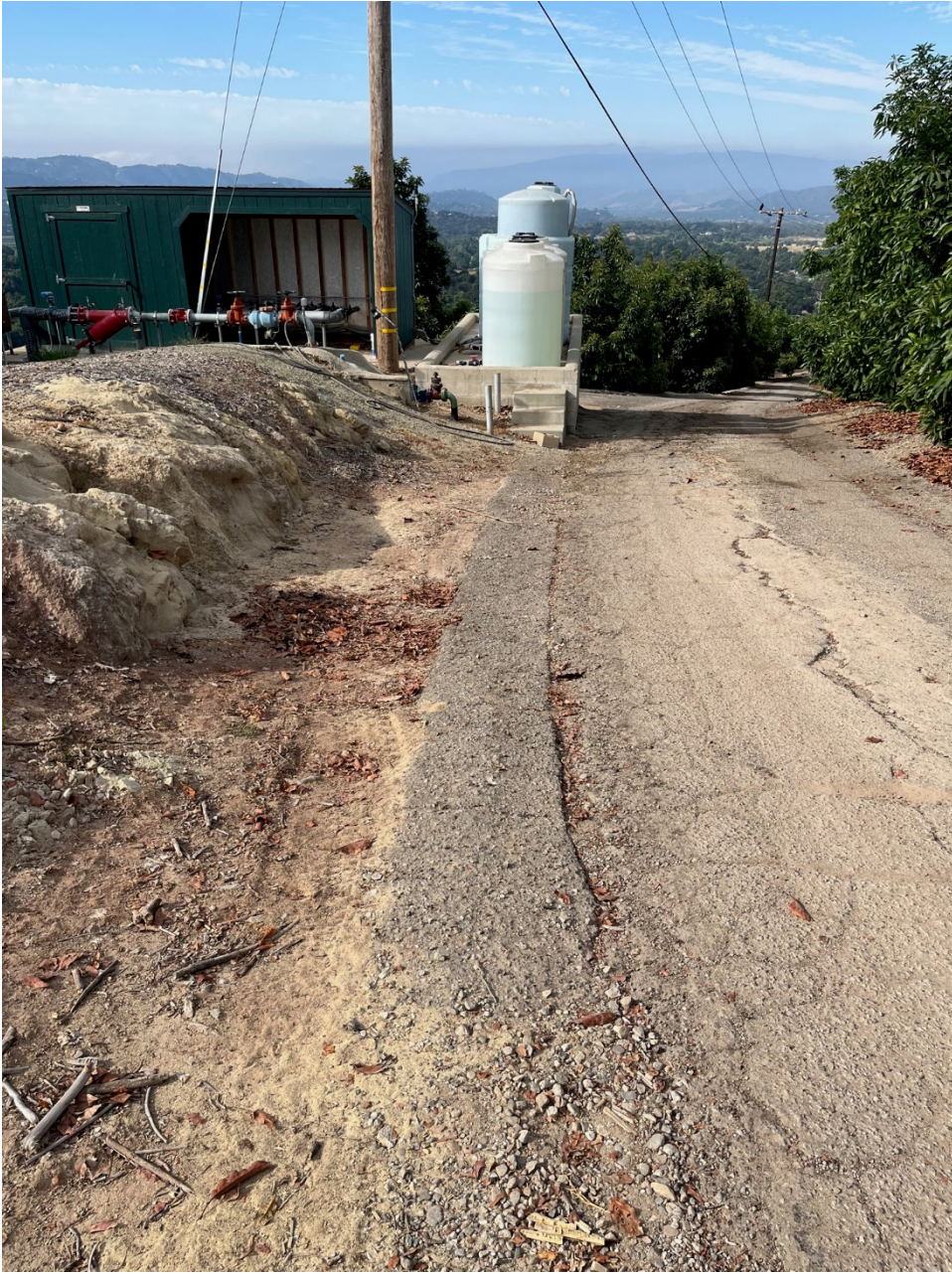
Upper Tank Site
