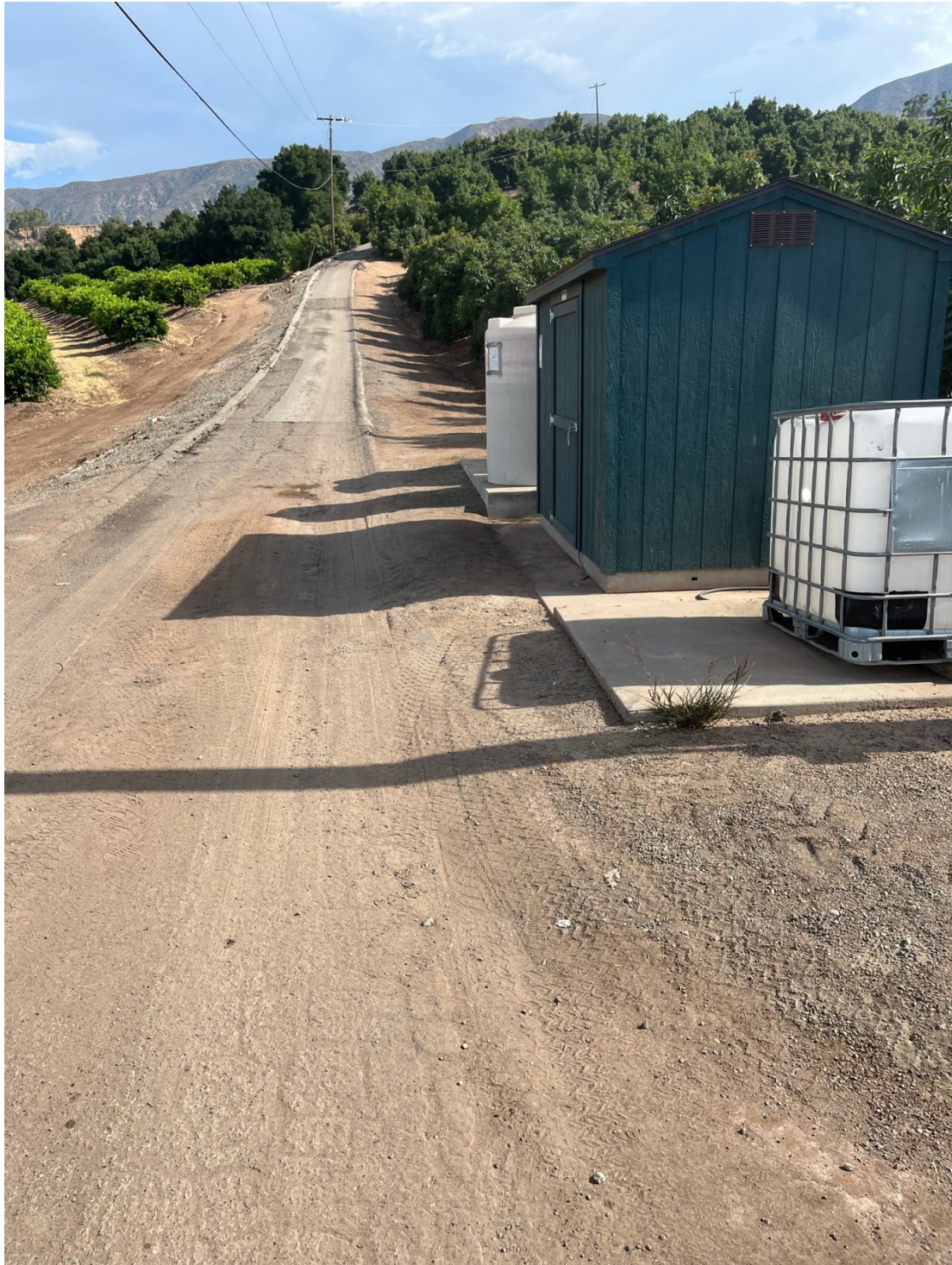
Lower Tank Site
