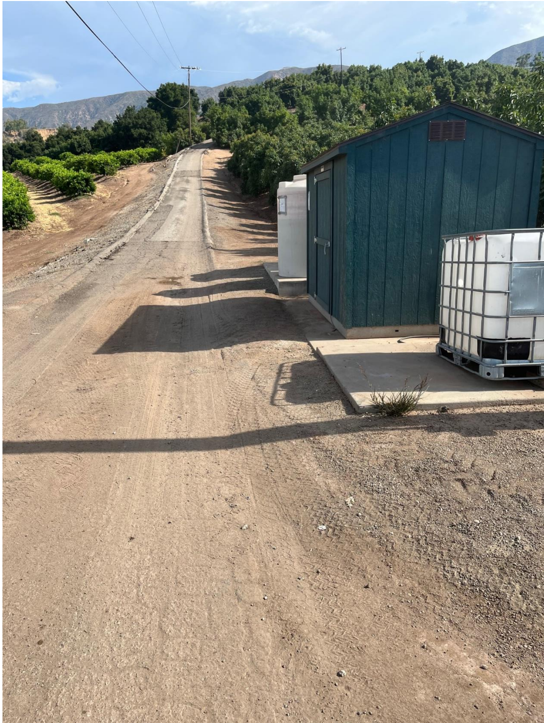
Lower Tank Site
