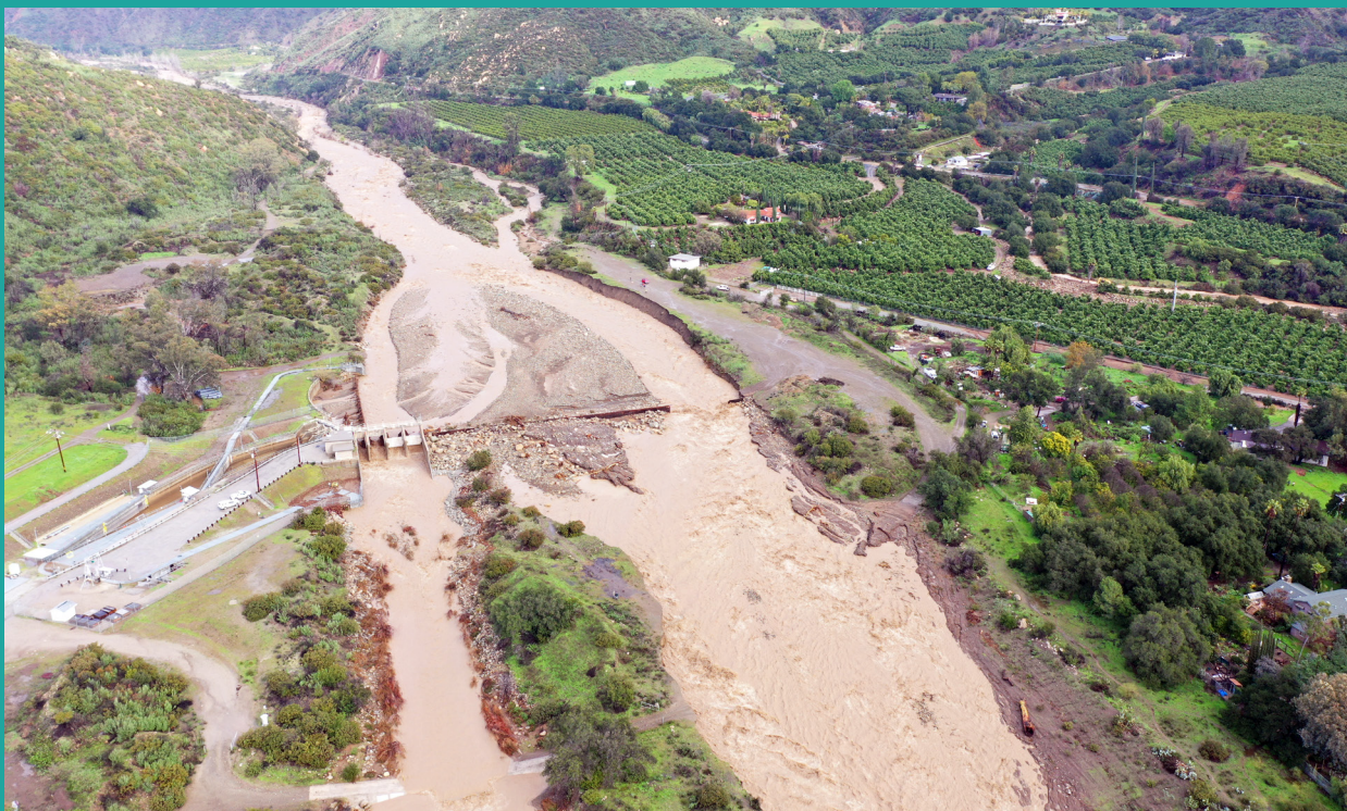
Photo above is from January 10, 2023 following the storm damage that occurred on January 9-10, 2023. The timber cutoff wall was breached on the eastern side causing flows to go around the diversion and fish passage structures, and the facility was filled with sediment and debris.
