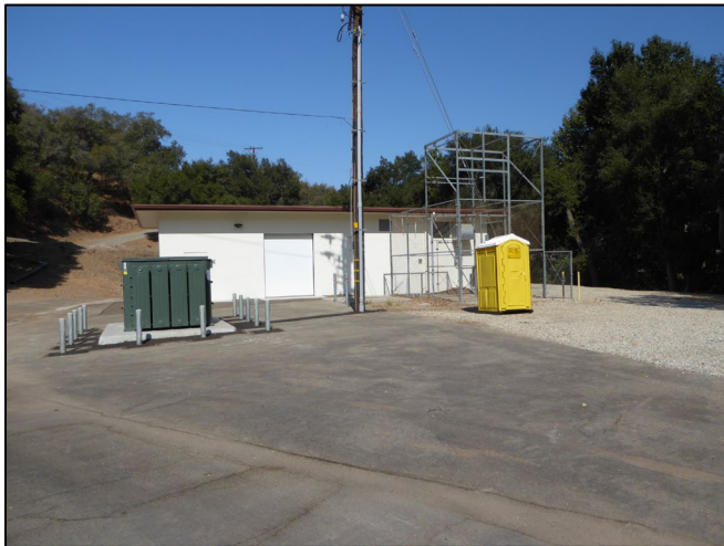
Rincon Pump Plant Electrical Building
