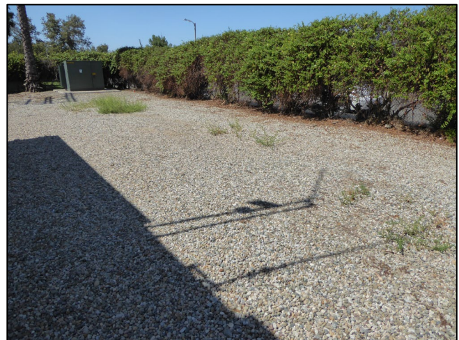
Proposed Generator Location At Avenue 2 Pump Plant
