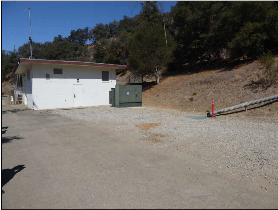
Avenue 1 Pump Plant Electrical Building and Proposed Generator Location
