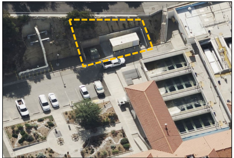
Aerial Photo of the Lenain Water Treatment Plant Generator Set
