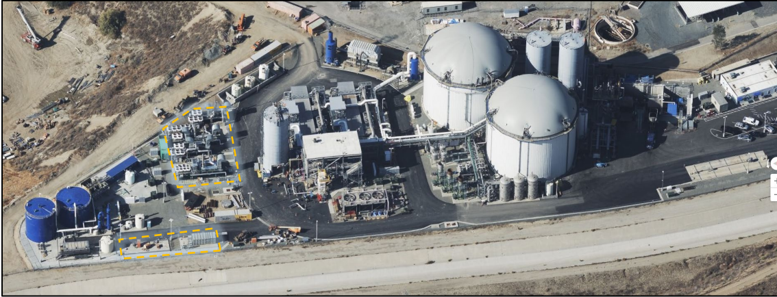
Aerial Photo of the Rialto Bioenergy Facility
