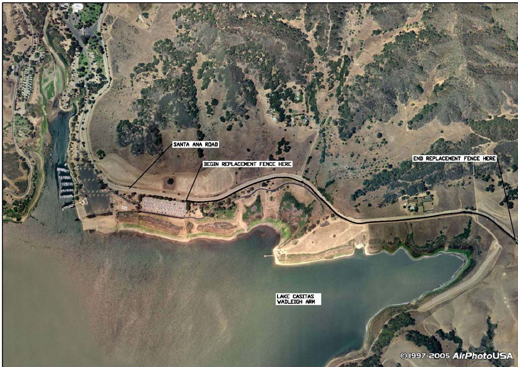
Figure 2. Overview of the fence replacement portion along Santa Ana Road
