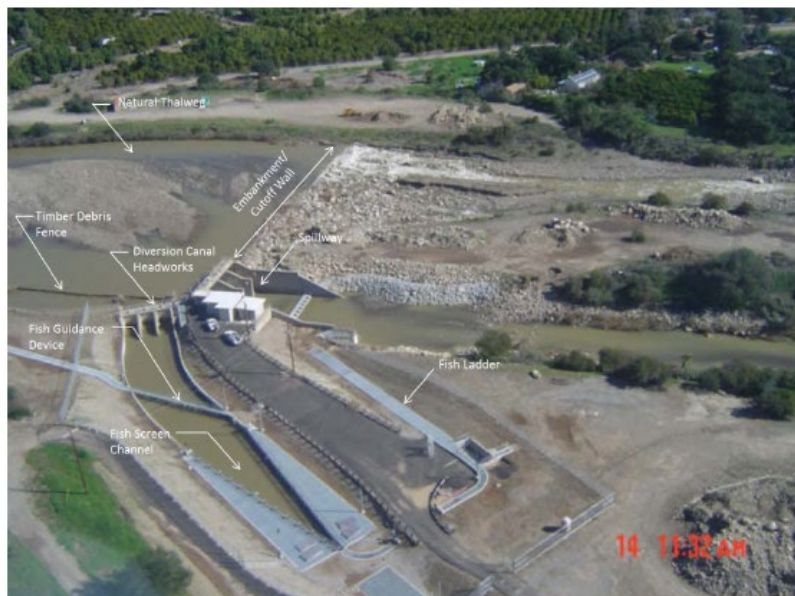
Figure 5-5. Robles Diversion Fish Screen (MKN Associates, 2019)
