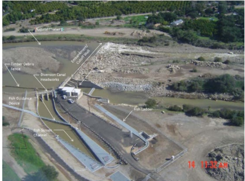
Figure 4-5. Robles Diversion Fish Screen (MKN Associates, 2019)
